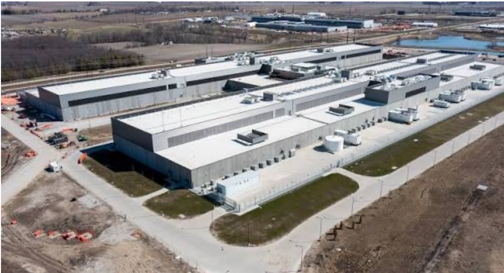
Polk County (FL) Data Center Image: Turner Construction Company
